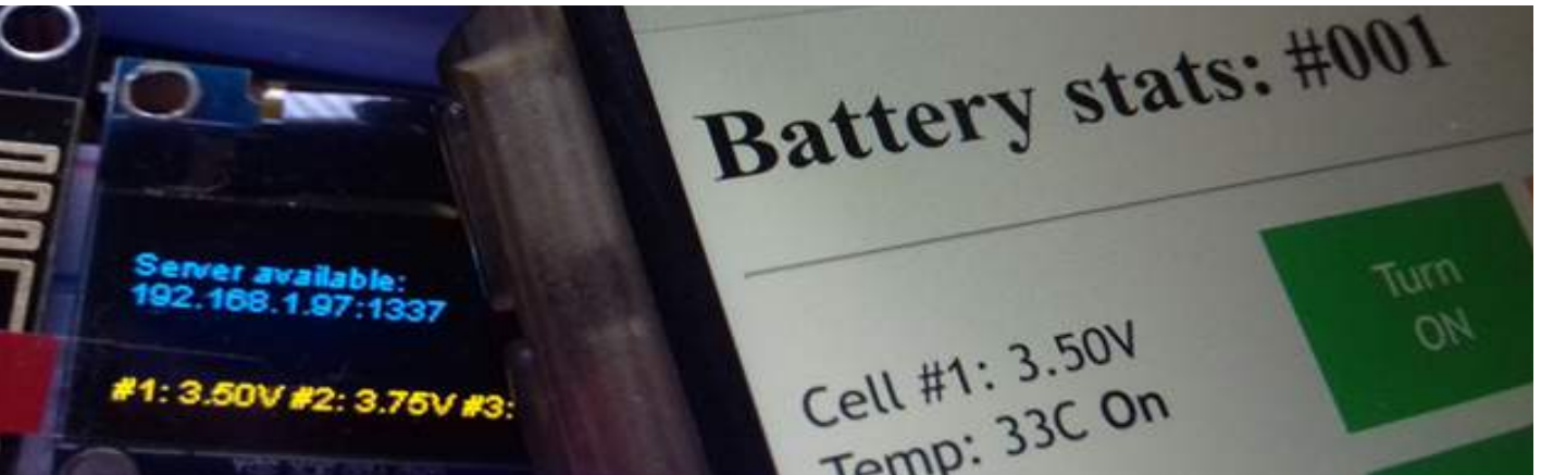
Figure 13: LCD showing IP address and battery insights, Web page showing available data about the battery
